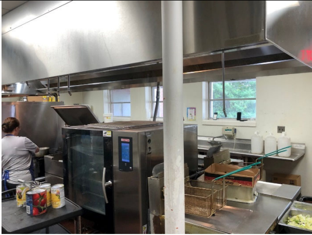
View of the Kitchen.
