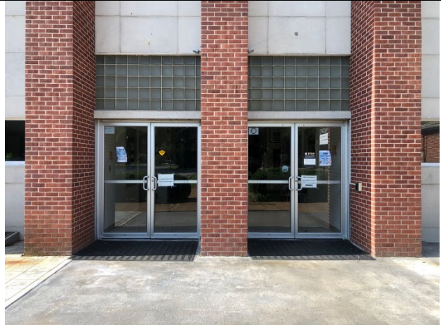
View of the Main Entrance.
