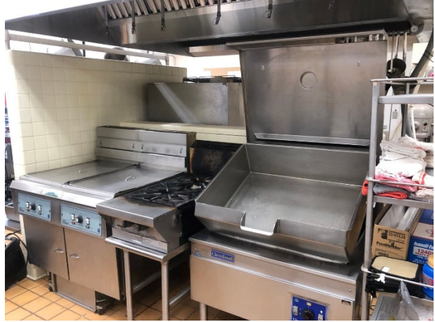
View of the Kitchen.
