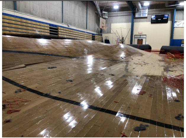
View of Athletic Flooring Damage.
