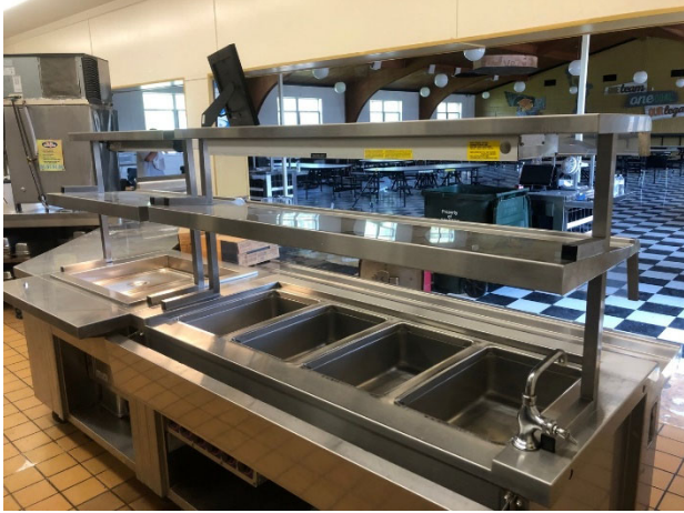
View of the Serving Line.
