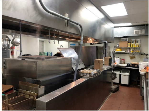
View of the Kitchen.
