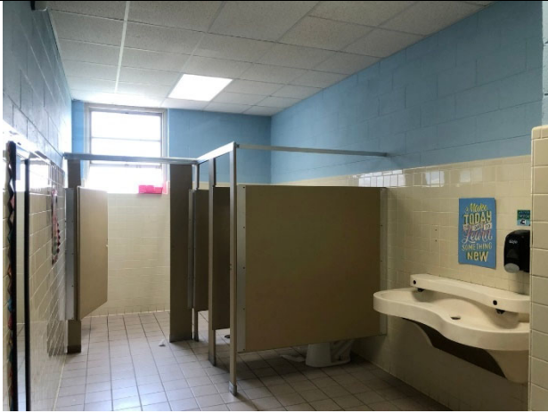
View of Restroom – Main Building.
