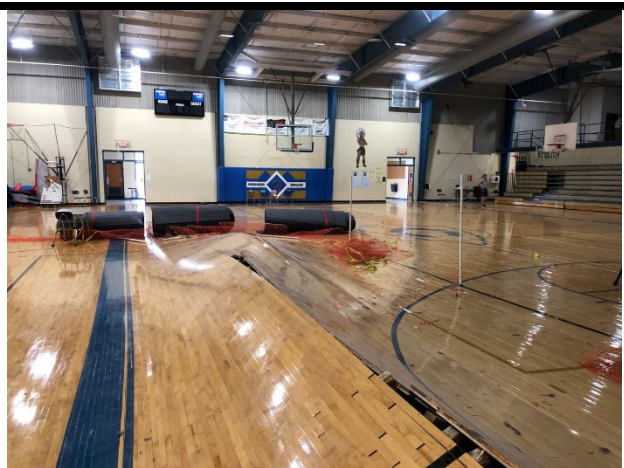
View of Athletic Flooring Damage.
