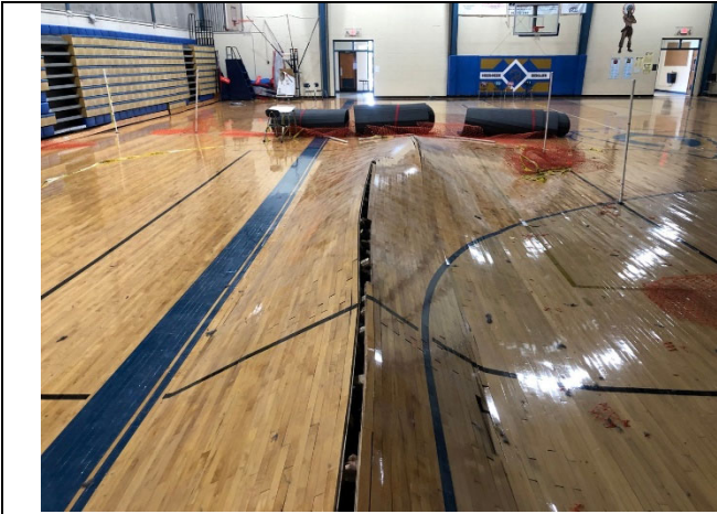
View of Athletic Flooring Damage.
