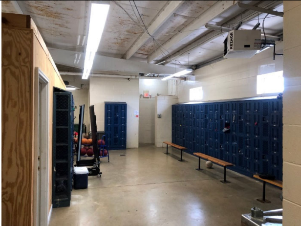
View of Locker Room.
