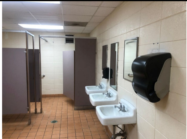
View of Restroom – Addition 'C'.
