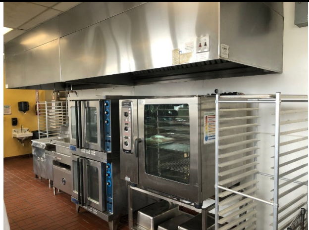
View of the Kitchen.
