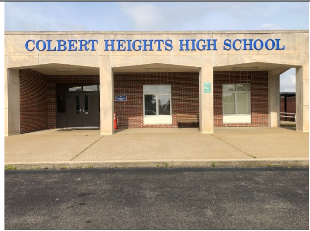
View of the Main Entrance.
