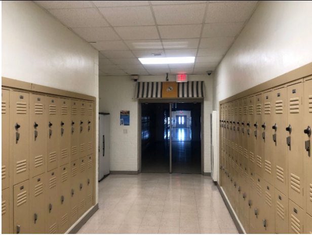
View of Corridor – Addition 'B'.
