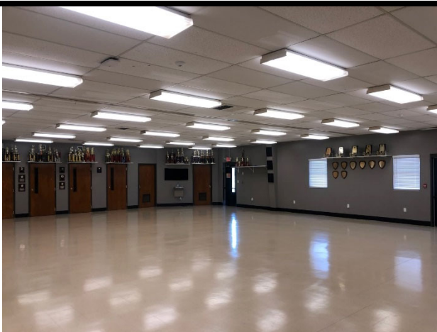
View of the Band Room.
