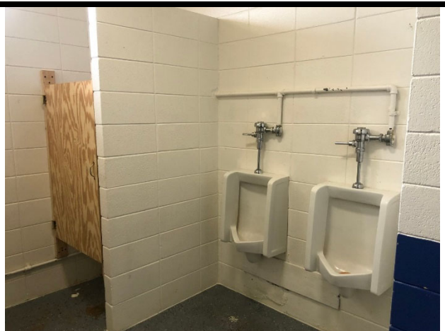
View of Locker Room Restroom.
