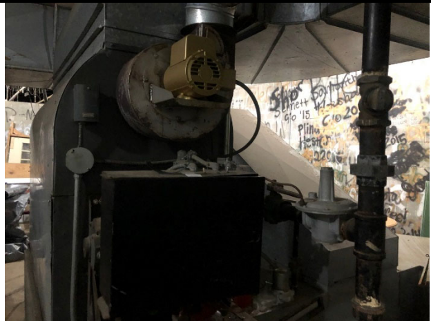
View of the Boiler Room (Auditorium).
