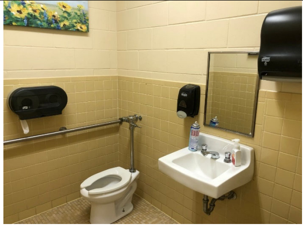
View of Restroom – 1979 Addition.
