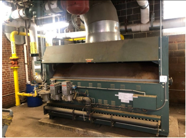
View of the Boiler Room.
