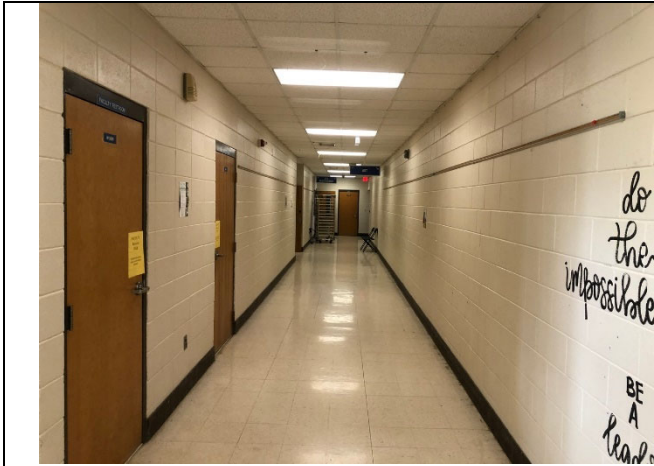
View of Corridor – 1995 Addition.
